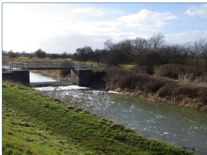
Before – Aubourn Weir showing the drop of approximately 1m which created a barrier to the passage of fish and eels
