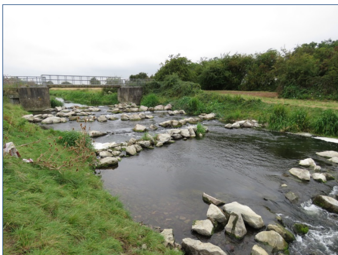
After – the completed Aubourn Rock Ramp fish pass. Fish and eels can now pass freely upstream and downstream
