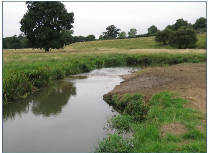
*After – New gravel riffle created to speed the flow and bank lowered to improve the floodplain connection*
