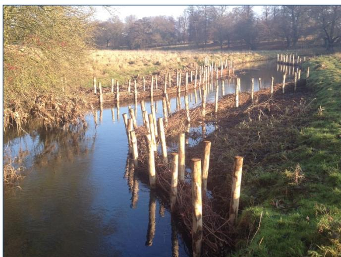
*Work in progress on a faggot-fronted berm to trap fine sediment, narrow the channel and speed up the flow*
